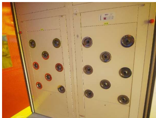
EQUIPPED WITH AN AIR SHOWER SYSTEM.
